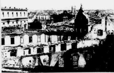
VIEW OF THE BURNT OUT RESIDENZ.
