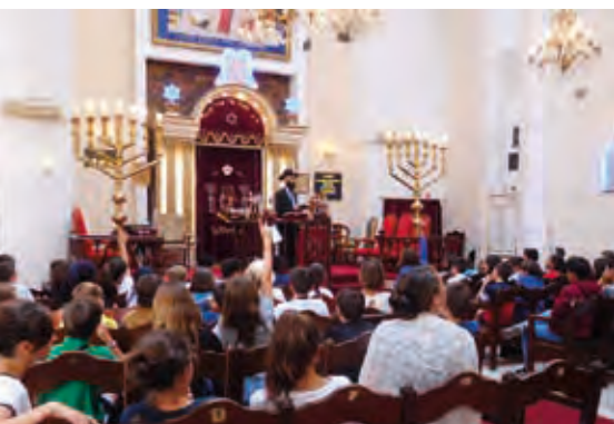
The Fund finances work to bring the electrical installation of the Bez Zakai complex in Montpellier up to code.
